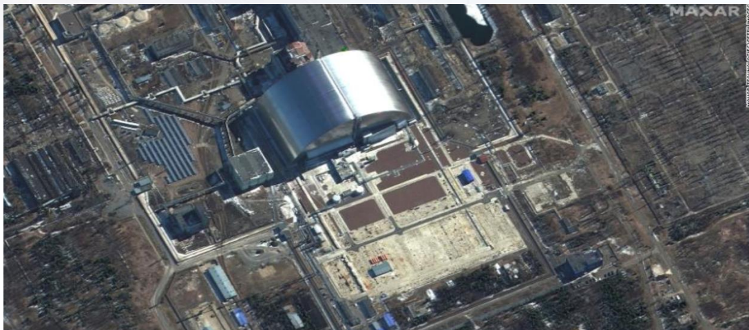
A satellite image of the power plant
